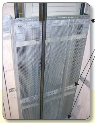
High form stability due to three surrounding brackets and 1.5mm thick galvanised perforated sheet panels.
