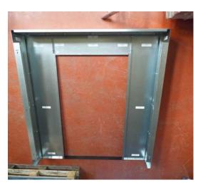
5. Connect the left (14), right (14) and top wall(13) panels to the three front panels (10),(11),(12)
