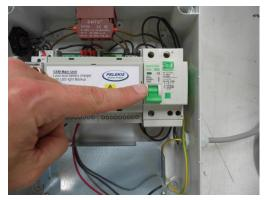
Connect the incoming main supply voltage: 230VAC to the power lead.
