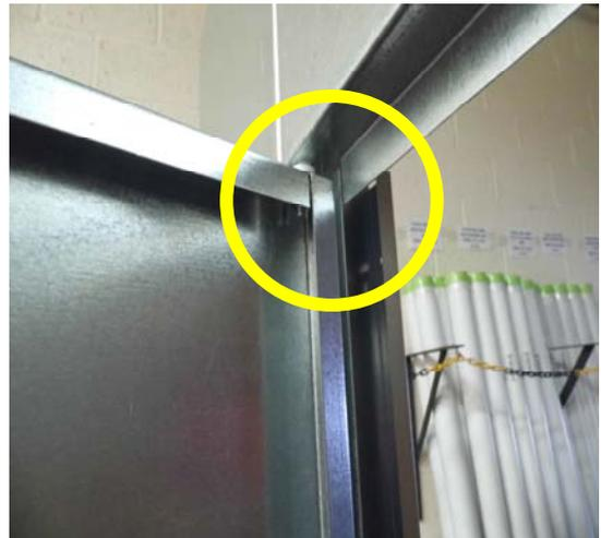
10. Position the top of the door in line with the top panel and insert M8 x 30 Cap Screw(16)
