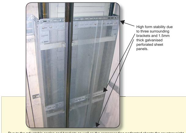
Due to the adjustable angles and brackets as well as the corresponding perforated sheets the counterweight cover virtually fits in every concrete lift shaft.
