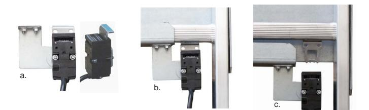
a. Fasten the switch to the switch plate (here exemplarily on the right). Insert the actuator so that its fixing bracket points to the back (in the direction of the shaft wall).
