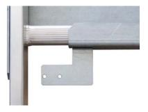
The switch plate has to be fixed according to the position of the ladder, on the far side of the shaft door.
