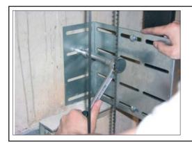
Fasten the first angle on the wall with dowels, flat washers and hexagonal wood screws.
