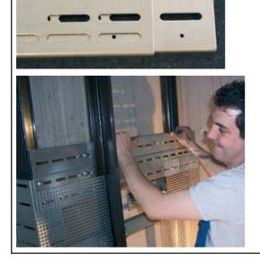
The panel mounting profiles middle/below (parts 4-1/2) can be telescoped. By applying on the upper mounting profiles (parts 3-1/2) the exact length is adjusted. The profile is screwed with two coach bolts M8x20.
