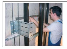
Transfer the mounting height of the angle with the water level on the other side.
