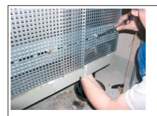
When all mounting angles are fastened, the remaining panels are assembled. Normally the panels overlap thereby.
