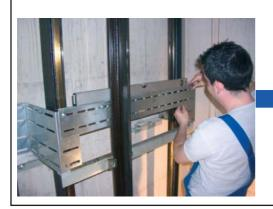
The fastening of the mounting profiles with each other is effected each with two coach bolts M8x20. The fastening with the mounting angles is effected each with one screw.
