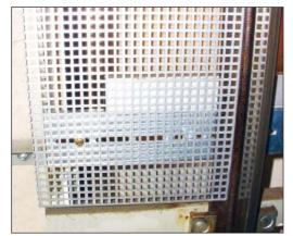
Fasten the lengthwise adjusted panel mounting profiles once centric and once below on the already assembled panels. Thereby the short sides of the profiles point to the counter-weight.
