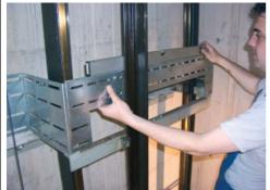
Lie the mounting profiles with the short side on the mounting angles.
