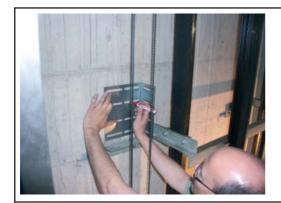
Hold the liftshaft wall sided angle on the wall. Thereby the upper edge has to lie 2.55m over the shaft ground. Mark a borehole in one of the vertical slotted holes. Drill the hole with a 12mm concrete drill.
