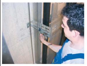
The second mounting angle is fastened in the liftshaft wall with dowel, flat washer and hexagonal wood screw.
