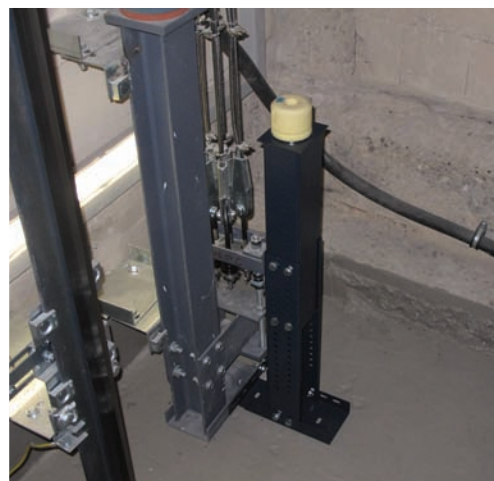
Mounting example buffer support size 4 with buffer
