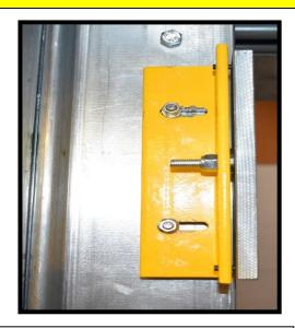
Position the Lock plate to the leading edge of the car shutter gate
